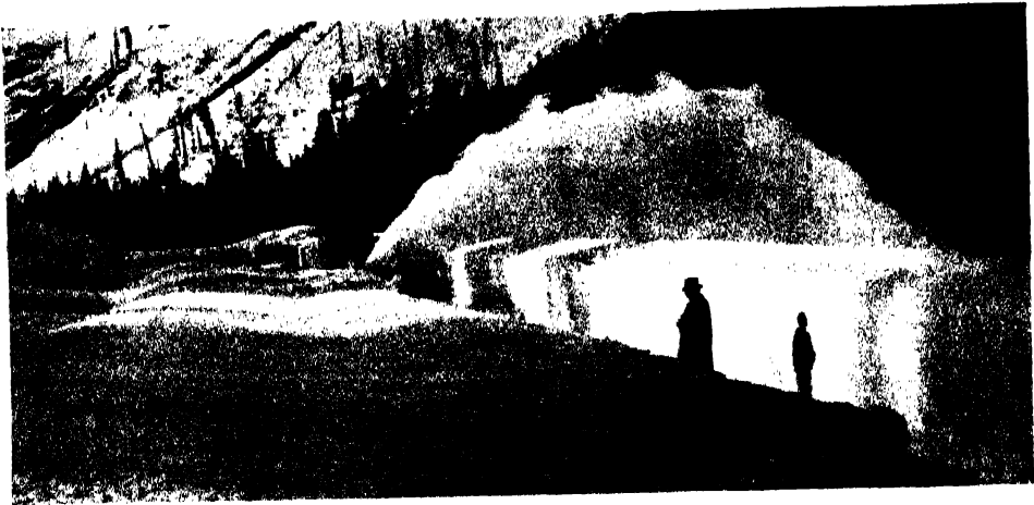
CUTTING A ROADWAY THROUGH STEVENS PASS IN WASHINGTON STATE AT THE END OF A WINTER SEASON.
